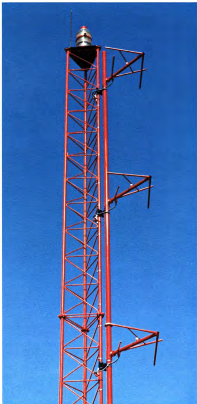
JAMPRO JSCP 3 bay shunt fed antenna using 3/8" rigid line. Note deicer cables.
