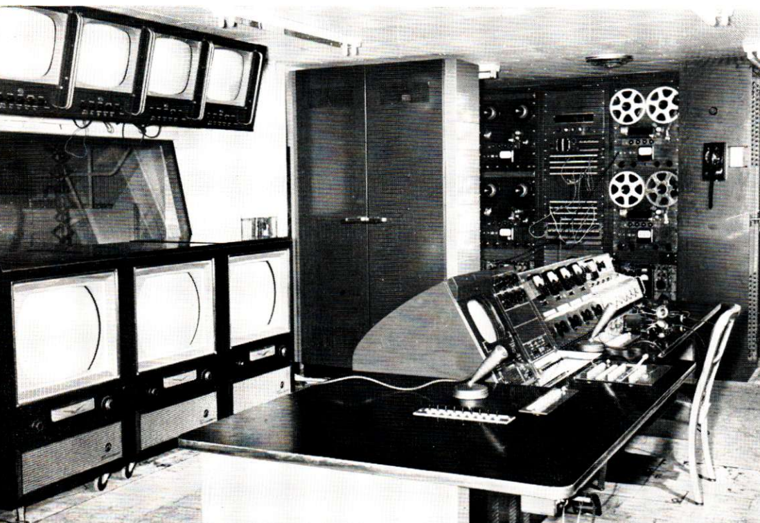
FIG. 3. Master control at AFIP. Programs from all three buildings are received and distributed from here. Window at left overlooks main studio.
