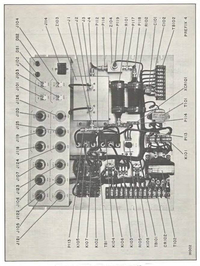
Figure 14. Exciter Switching Relay Panel, Rear View
