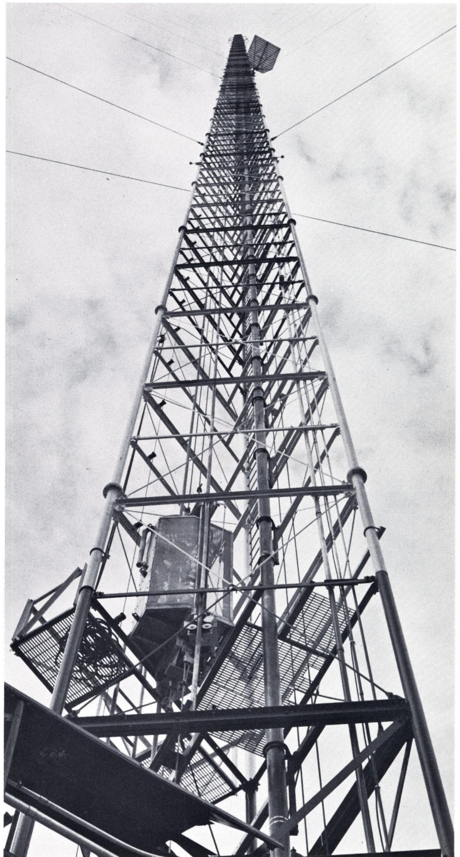
Vertical run of transmission line inside a triangular cross-section tower. Spring-tensioned hangers allow movement of the line due to thermal expansion and contraction.
