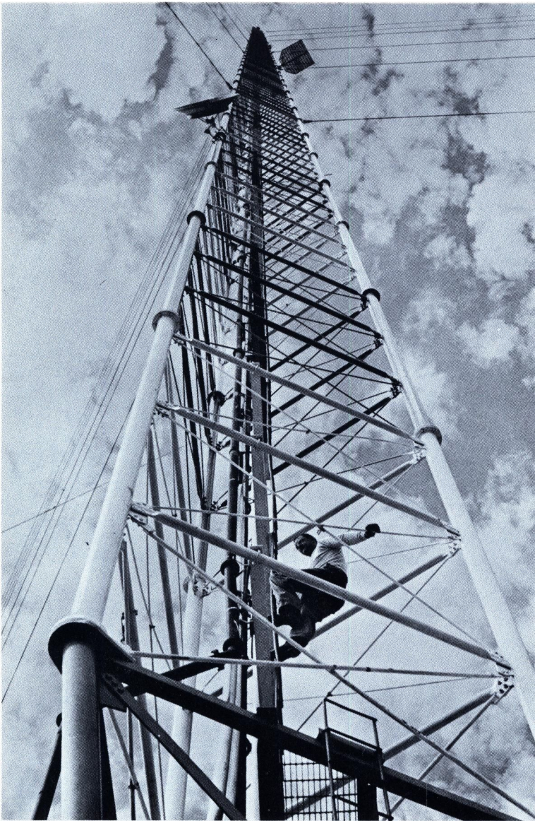
Guyed television towers can achieve great height at less cost than self-supporting structures where land value is not a determining factor. Towers are triangular and are available with either fixed or pivoted base.
