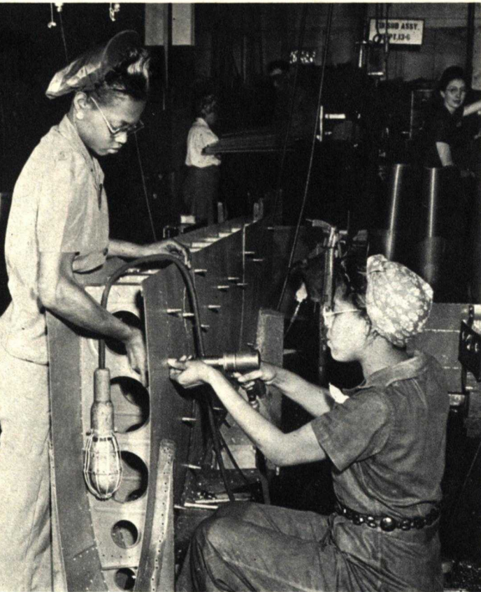
The "skin" (aluminum covering), held in place by skin fasteners, is riveted to the stabilizer by workers.
