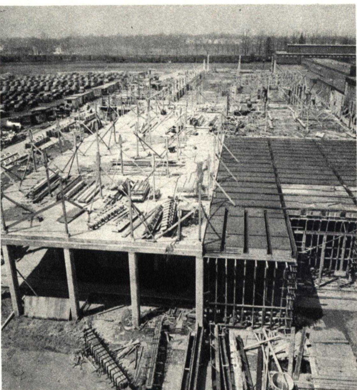
Trenton's final assembly line needed more room to meet higher schedules. Problem was solved by this addition.
