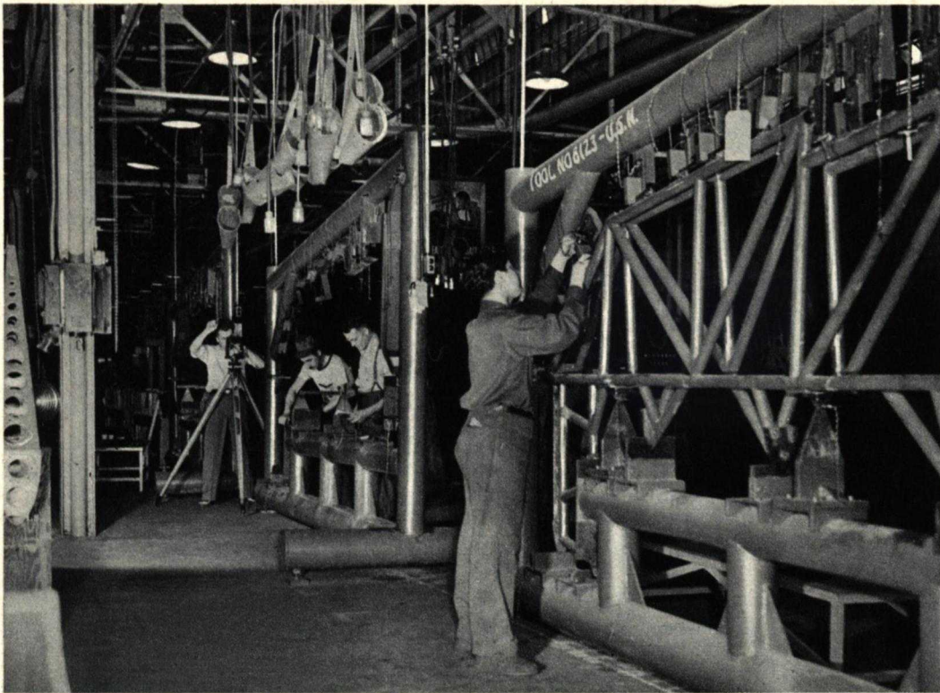
Special aircraft jigs and fixtures were installed and then tested for accuracy.
