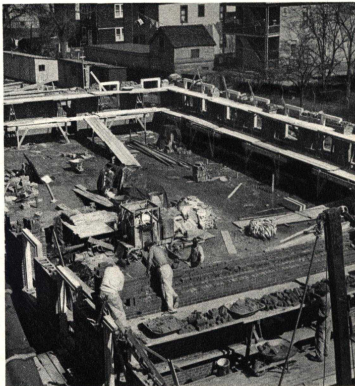
More space was needed at Bloomfield. High brick walls frame a new large addition to the main Bloomfield plant.
