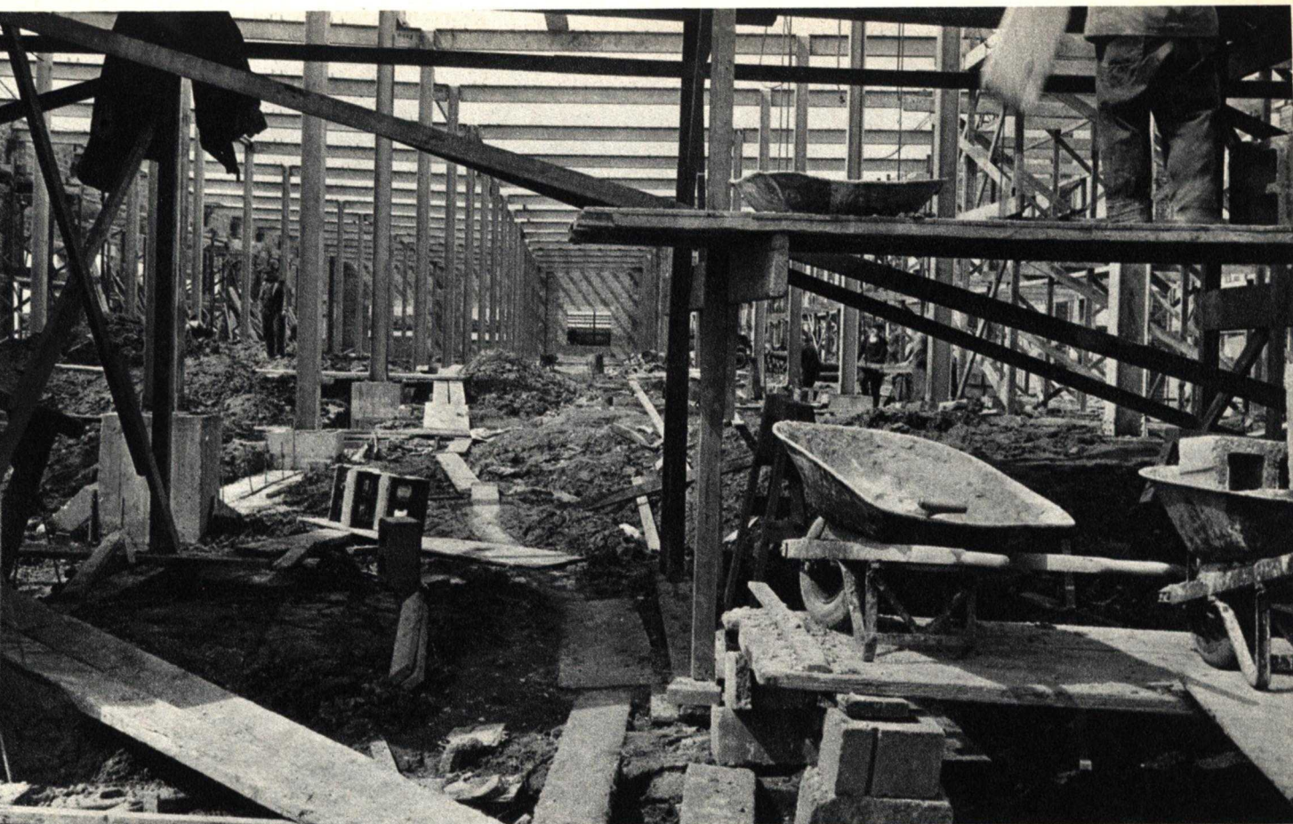
A labyrinth of lumber, steel and concrete forms into another new building at the rear of the Linden plant. The packaging, classification and shipping of Wildcat spare parts necessitated this vast, new addition.
