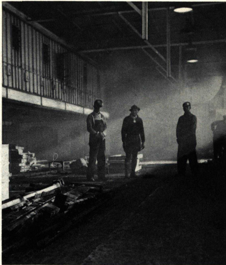
Out went the fixtures.
