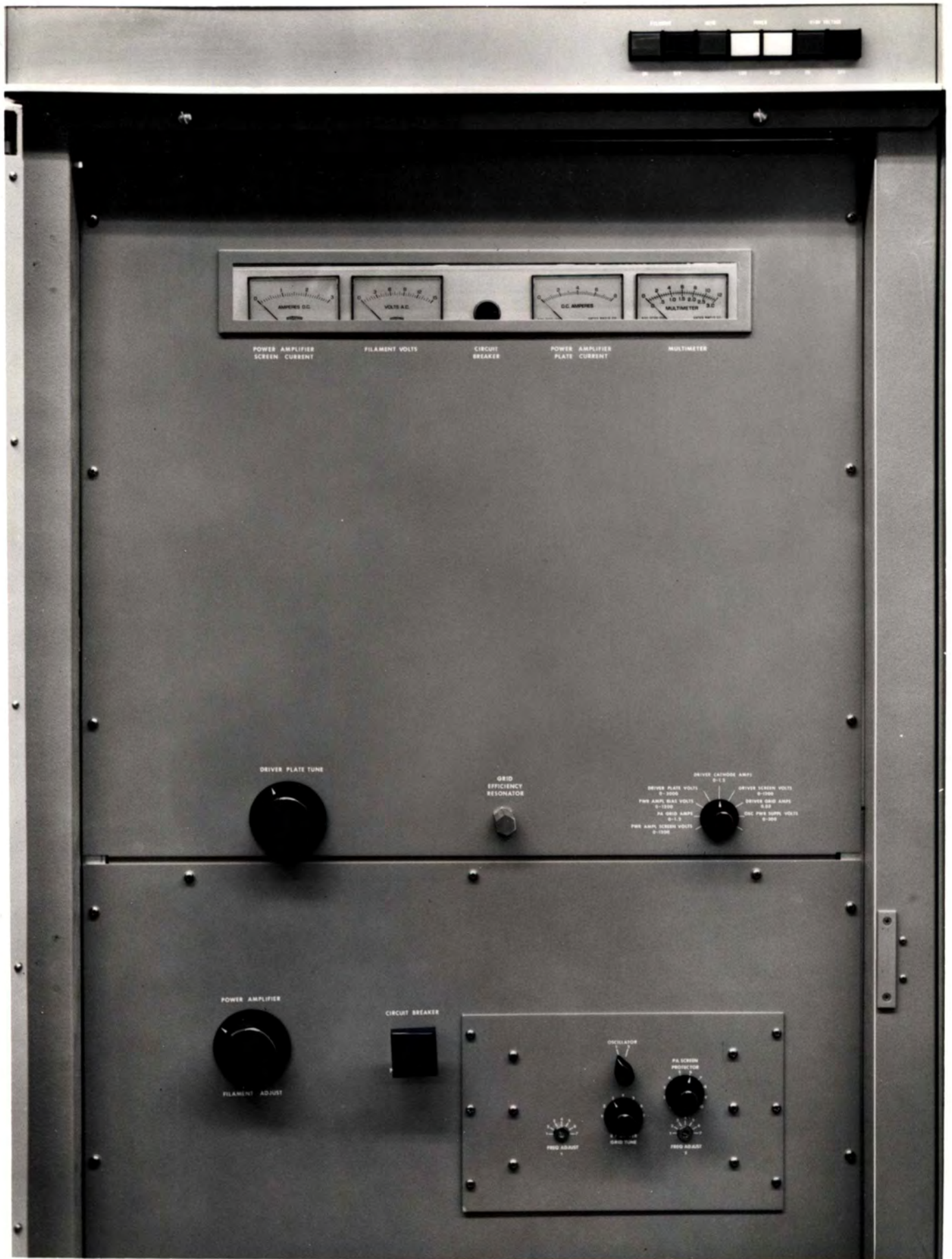
FRONT VIEW OF GATES' MW-50 RF CUBICLE, SHOWING DUAL OSCILLATOR CONTROLS AND ISOLATED METERING. 1891
