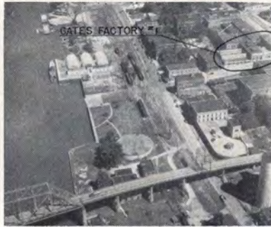
Gates Plant No. 1 On Mississippi
