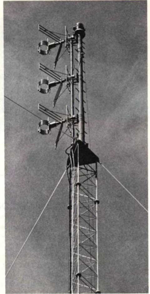
(Left) WGEM-FM, Quincy, Illinois utilizes a Gates 9-bay Dual Cycloid Antenna, leg mounted on the WGEM-TV tower. The top four bays are shown during installation.
