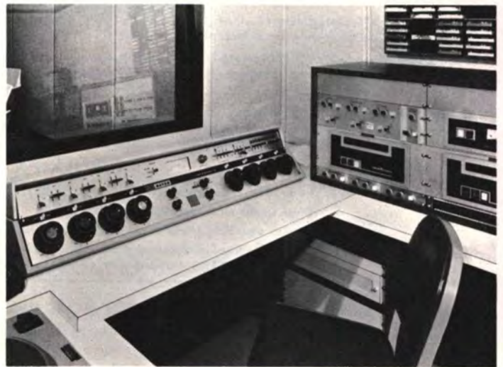
GATESWAY II CONSOLE AND CARTRIDGE TAPE EQUIPMENT WEEI, BOSTON
