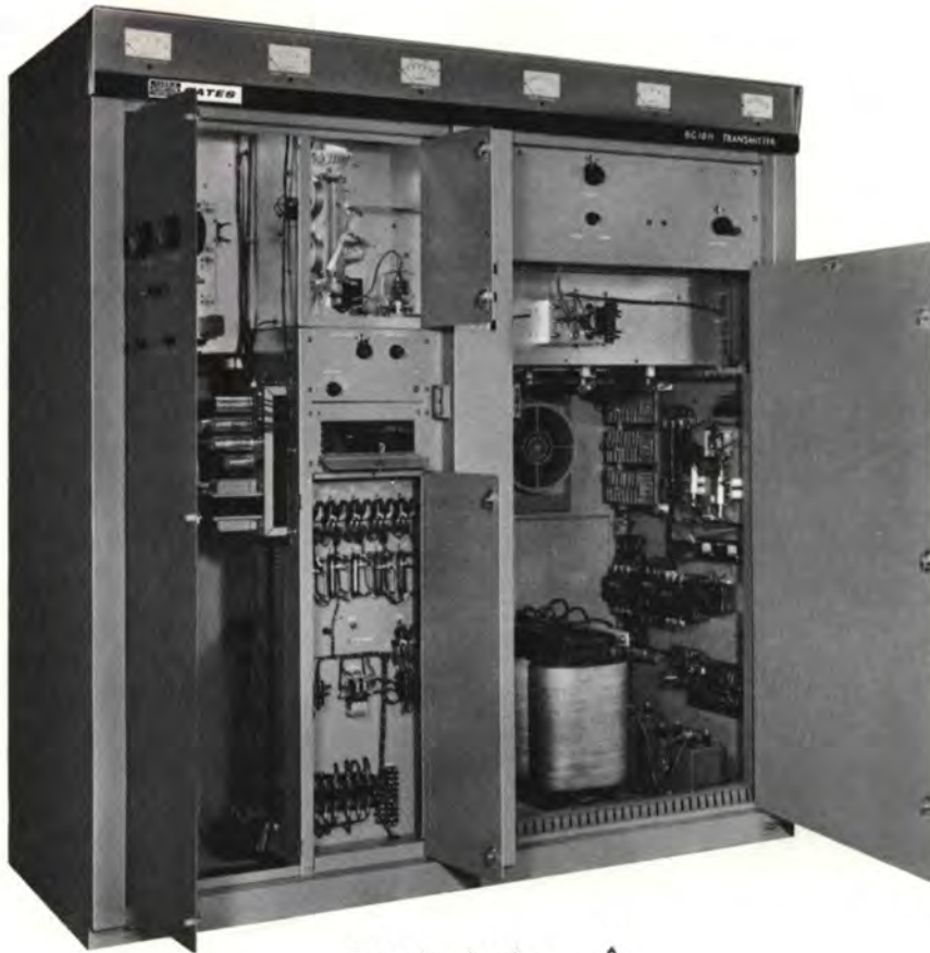
Front view, interior.
