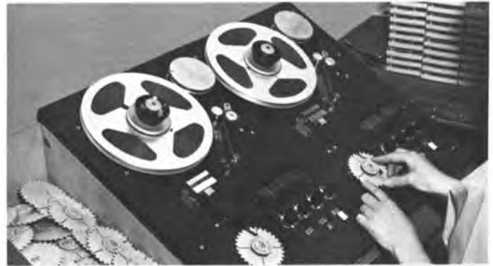
Tape is wound onto cartridge turntables with a precision tape winding machine to assure exact tape length and playing time.
