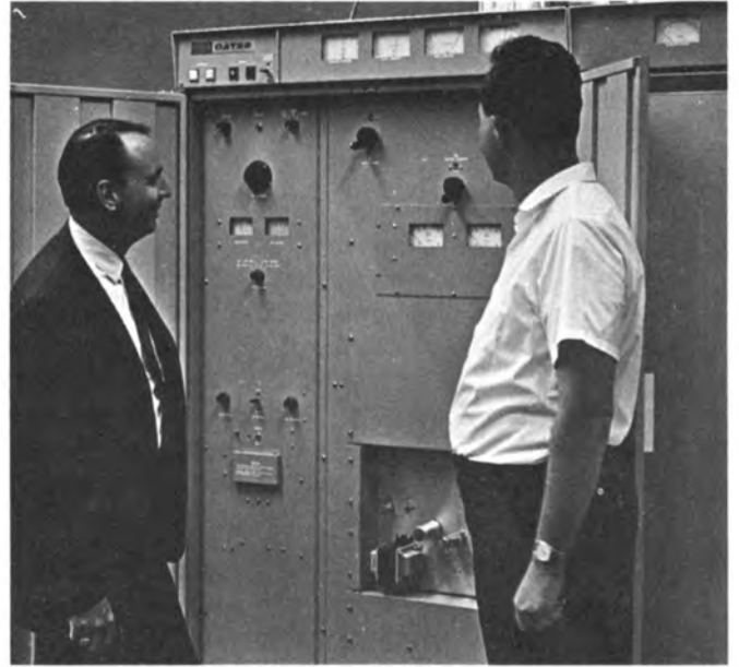
WGAN-FM, PORTLAND, MAINE —Utilizes a Gates 40 kW FM transmitter (two 20 kW transmitters with combiner and common exciter).
