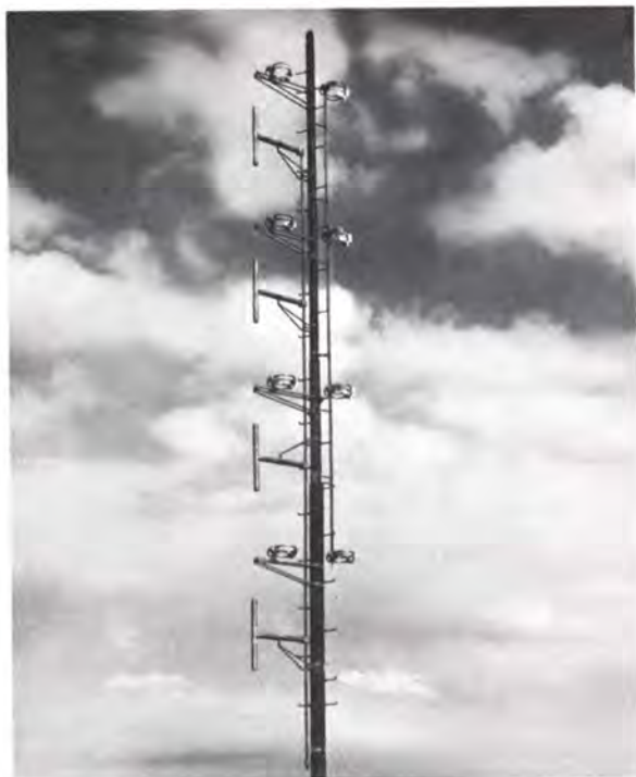
Directional FM antenna as supplied by Gates to Radio Station WMSH, Hershey, Pennsylvania. Antenna consists of four bays directional Cycloid and four bays non-directional 300G elements.
