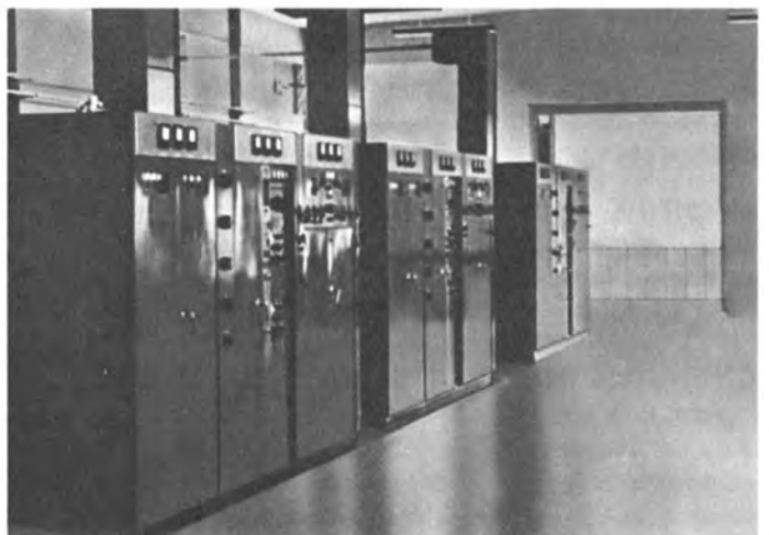
RADIO MALAYSIA —Three 100,000 watt short wave broadcast transmitters Model HF-100 now in operation at Kuala Lumpur.
