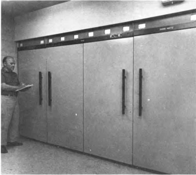
KDAY, LOS ANGELES —The first station to employ Gates VP-50 Vapor Cooled 50,000 watt AM transmitter.
