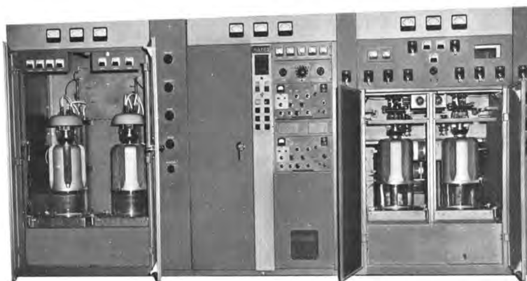
Three main transmitter cubicles house (from left to right) the modulator, transmitter control circuitry, and RF power amplifier.
