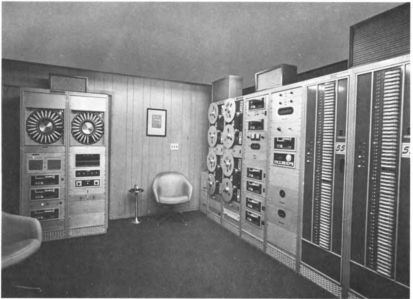
A complete broadcast automation system in the Automatic Tape Control demonstration room gives visitors a chance to see and hear automation in actual operation.
