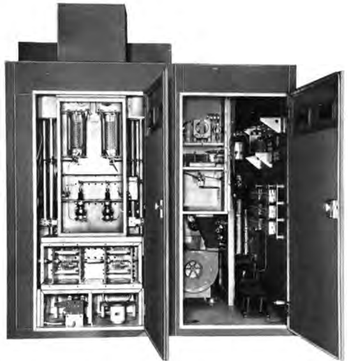
Rear view of PA and RF driver/exciter cubicle.
