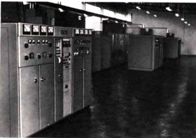
RADIO SINGAPORE—Three Gates 50,000 watt transmitters Model HF-50C used for high power short wave broadcasting. Note the outstanding installation arrangement.
