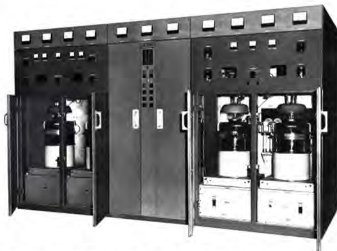
Three main transmitter cubicles house (from left to right) the modulator, RF driver, and power amplifier.
