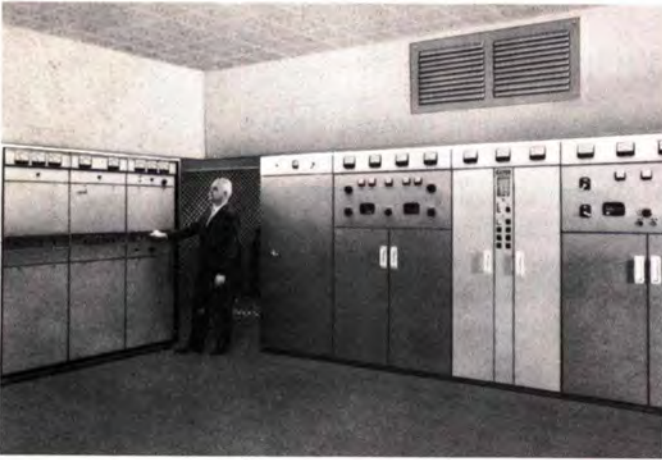
WIBC—INDIANAPOLIS—50,000 watt Model BC-50C and 10,000 watt Model BC-10P transmitters in this ultra-modern installation.
