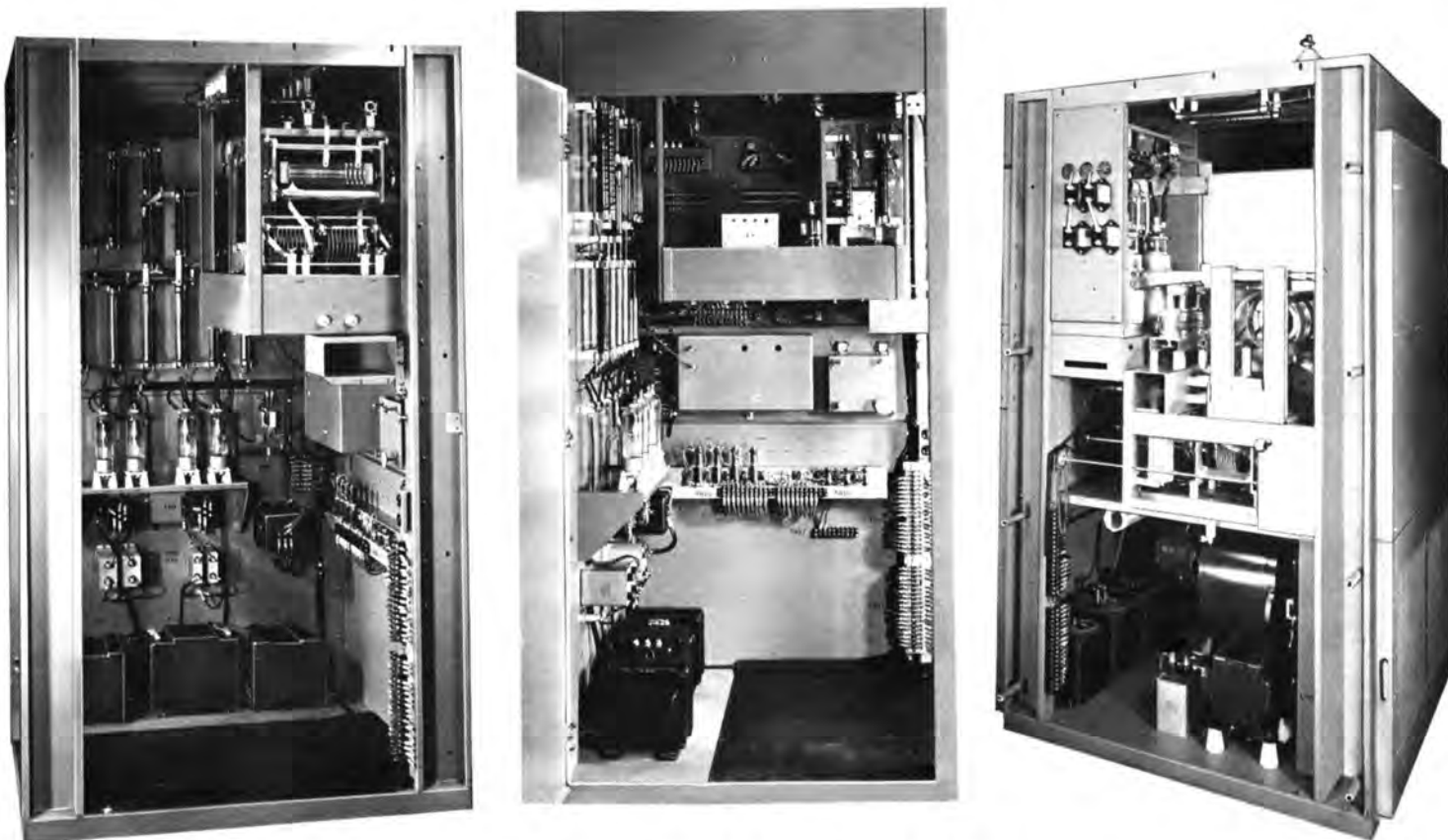
Rear view front left to right of RF drive cubicles and RF power amplifier center cubicle.
