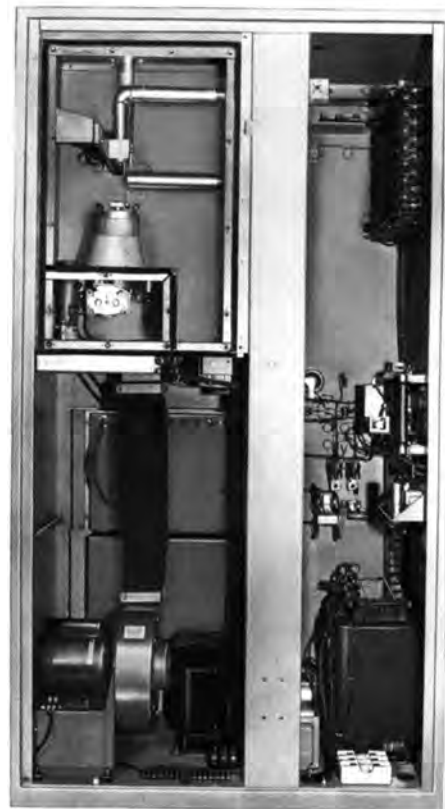
Accessibility, logical design and excellent workmanship are all illustrated in this back view with door and power amplifier panel removed.
