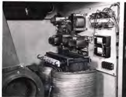
Power supply assembly (bias, screen and plate) can be reached quickly. Husky transformers invite 24-hour schedules.
