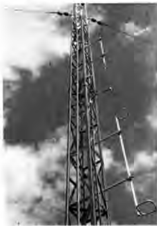
RA-4 Base Station Antenna.
