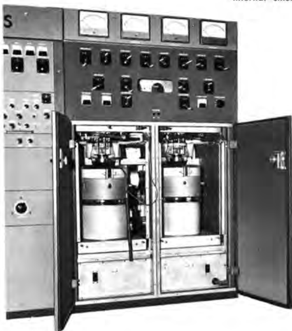
Front view PA cubicle with internal shields removed.
