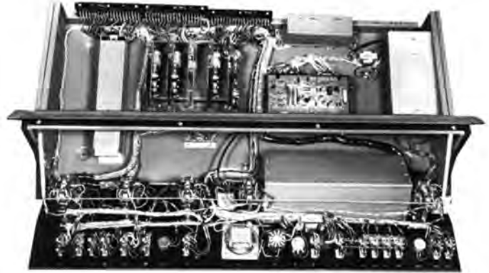
The smooth and easy to service design combined with the smaller size of transistorized components is best evidenced by the open view above. Note the plug-in amplifiers to the left, cue intercom speaker near center front and hinge down front panel and hinge up cabinet cover. "Control Center" is the shielded portion to the right of the cue speaker.
