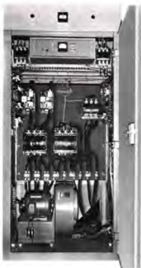
Front view of power amplifier contactor and rectifier cubicle. Note the husky AC contactors and the control unit for the regulated filament supply. A similar assembly is used for the modulator.
