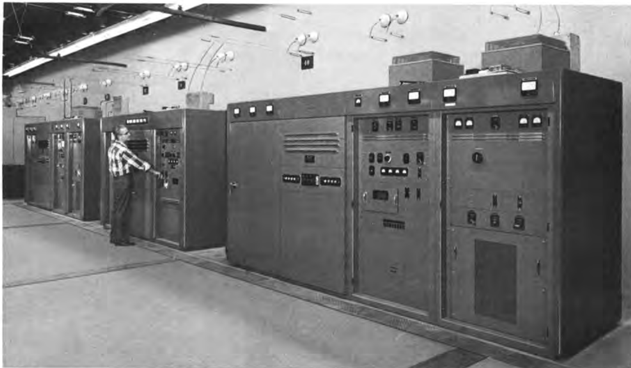
Two of Six Gates Model HF-10TX transmitters along with the 30KW model in continuous operation at the Press Wireless Transmission Center, Centereach, Long Island.
