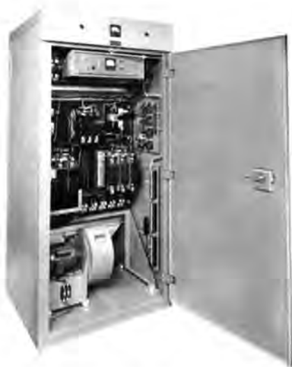
Front view of HV and AC contactor cabinet. Note electronic filament regulator.
