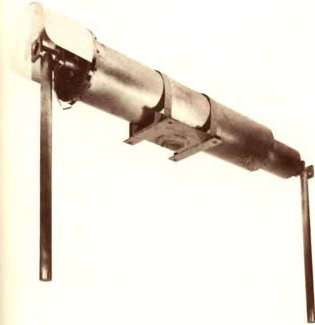
403-403A Isolation Transformers
