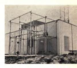
ing the main transmitter, dummy antenna, antenna network, auxiliary transmitter, transformer vault, and auxiliary generator. Note the equipment layout is functional; no effort has been made to dress up the plant or isolate the control area from the equipment. This plant joined our remote control family on April 12, 1961.
