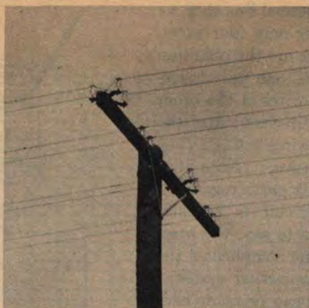
TRANSPOSITIONS IN 8-INCH SPACED OPEN WIRE LINE USING POINT-TYPE FIXTURES
