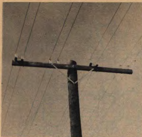
TRANSPOSITIONS IN 8-INCH SPACED OPEN WIRE LINE USING POINT-TYPE FIXTURES
