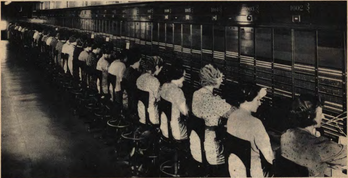
OUTWARD LONG DISTANCE SWITCHBOARD
