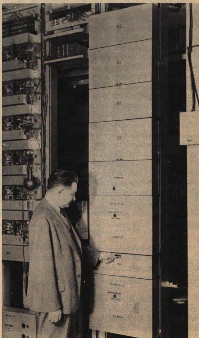
TYPE-K CARRIER SUPPLY BAY
