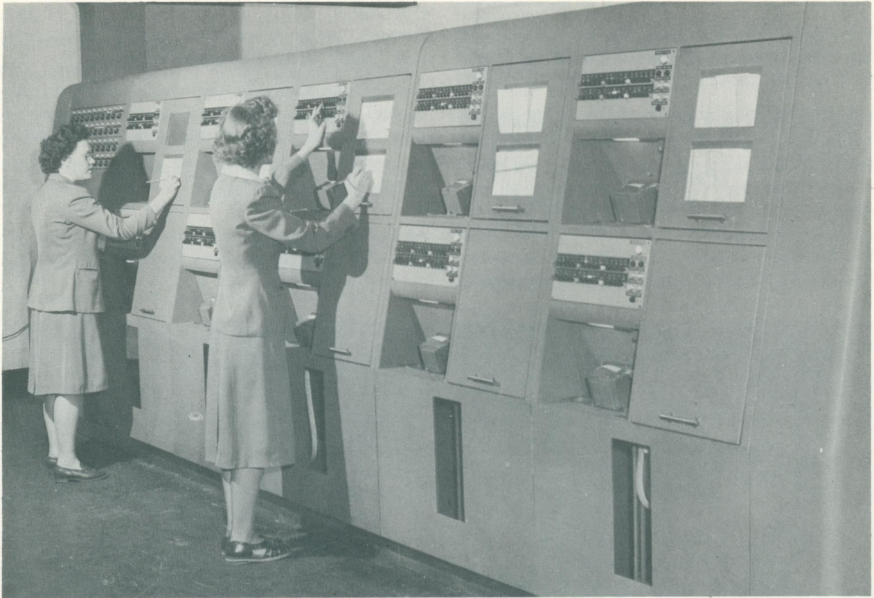
This is a bank of message switching machines in a Communications center. By pushing a button, operators can transmit messages to any station along the line's routes. Photo courtesy United Air Lines.
