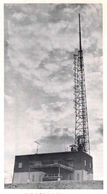
Vertical Polarized Antenna array.
