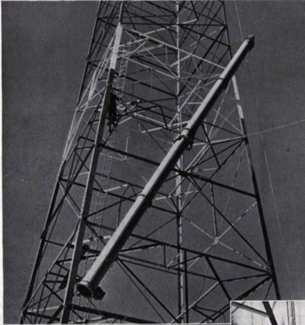
Raising the four-section Pylon in one completely assembled unit at WJPG-FM, Green Bay, Wisc.
