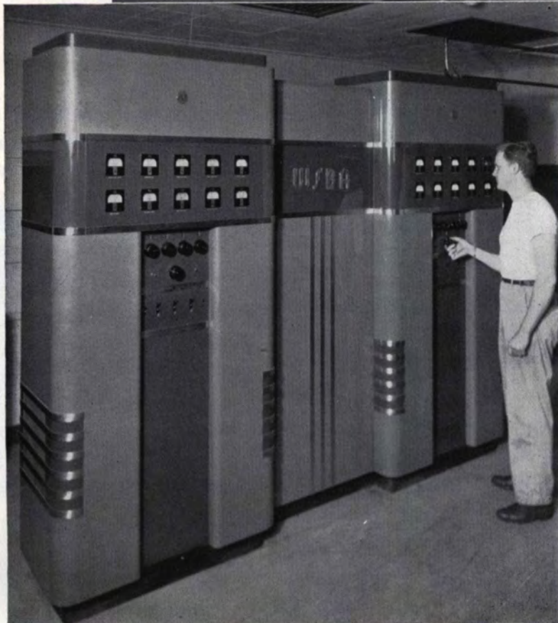
▲ Fifty kilowatt transmitter, Type BTA-50F, with control console and extension cabinets containing phasing equipment, at KMPC, Hollywood, Cal.
