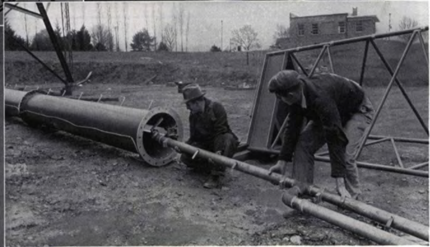
Inserting the transmission line harness into the two-section Pylon at WSBA-FM, York, Pa.
