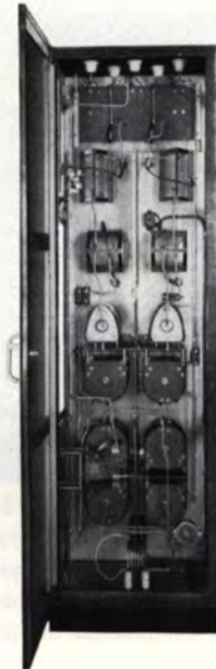
Interior view of a 1 KW phasing and branching equipment
