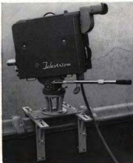
Parapet Clamp Support, MI-26189, as used with Hi-Hat to support RCA Field Camera
