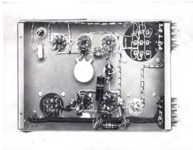
View of BA-12A Utility Amplifier Chassis showing component wiring
