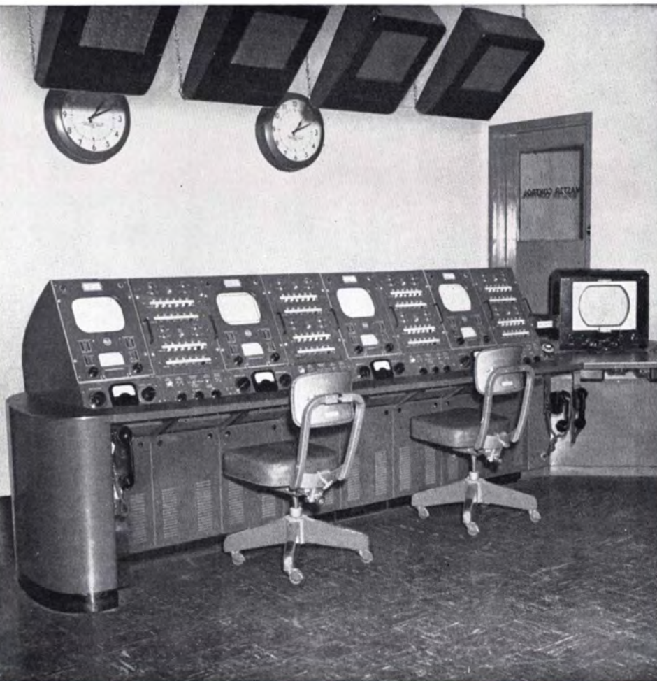
The studio console design shown above employs varied colored knobs and switch handles for easy and quick identification of individual controls. All escutcheons and dial plates are of attractive, long-wearing nickel silver.
