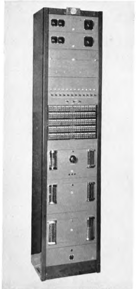
Line Terminating Rack at WHBC, Canton, Ohio.
