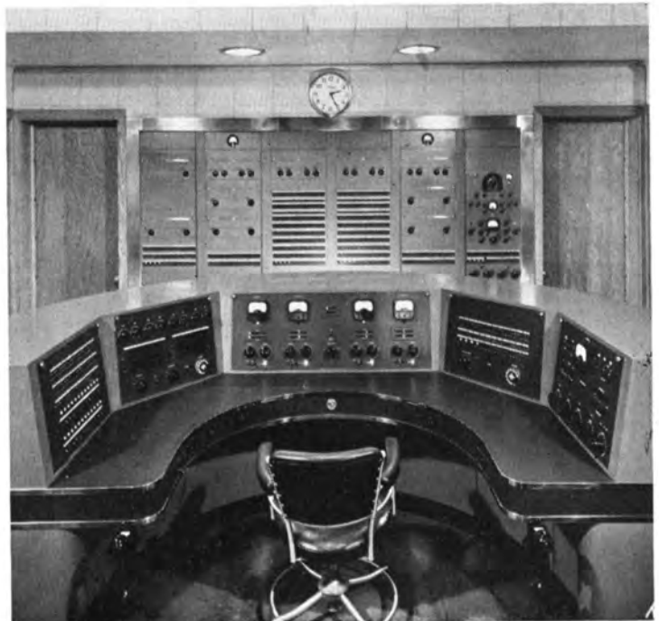
Master Control Room Speech Input of WLS.
