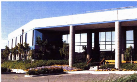
Pacific Research & Engineering Corporate Headquarters Carlsbad, CA
