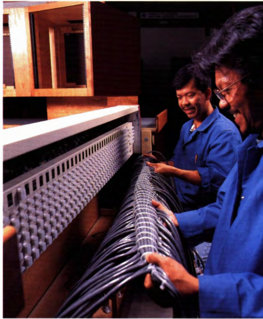
Experienced system assemblers install the pre-fabricated audio and control wiring.
