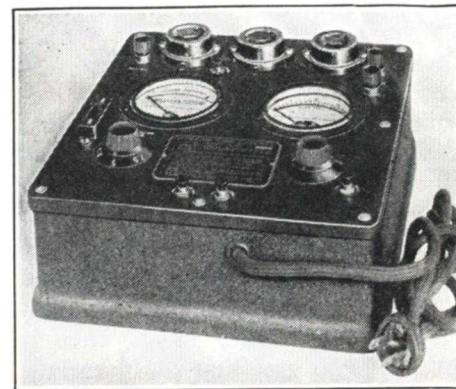
One of the first grid shift or mutual conductance testers designed for servicemen.
