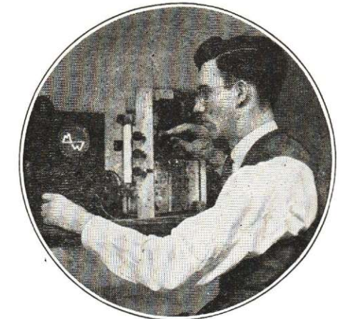
Using a cathode ray oscilloscope to see how the a.f. signal voltage in a radio set is varying.
