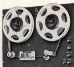
SPECIAL PURPOSE TAPE TRANSPORT USING 1-INCH TAPE ON 8-INCH REELS
