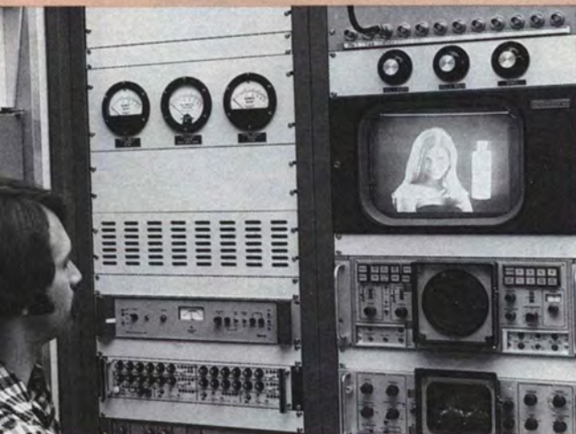
This TT50FL dual transmitter installation at WKYC-TV is the first in the country. Shown above are three TERMALINE "Reject Loads" with their THRULINE Wattmeters. The 50kW Test Load/Wattmeter above left is switched remotely (including water flow) from the studio 10 miles distant, where the reject power levels and main feed power are monitored (left).
