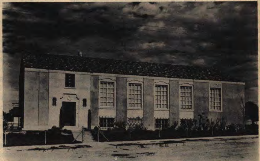
OPEN WIRE REPEATER STATION AT KINGMAN, ARIZONA
