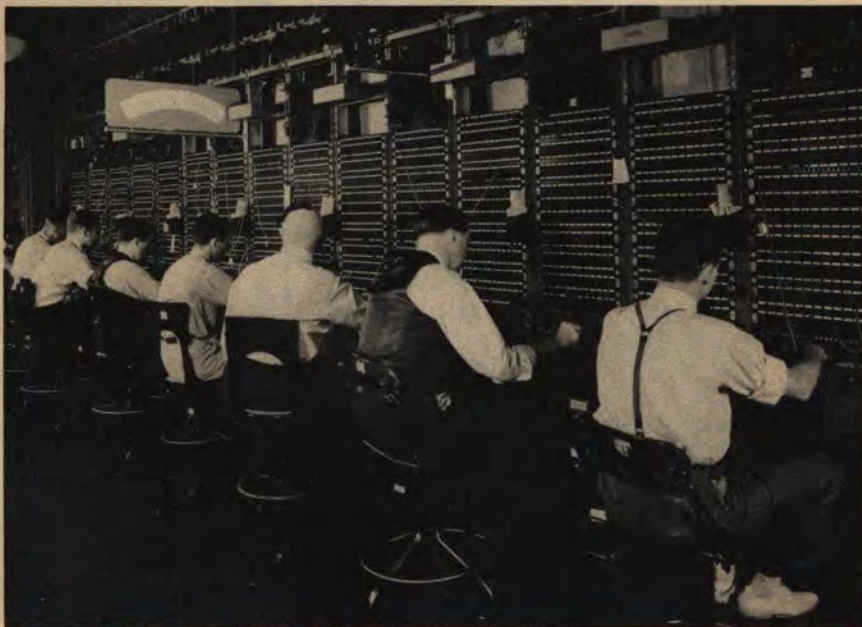
SECONDARY TOLL TESTBOARD SHOWING PROJECTION METER FOR TRANSMISSION MEASUREMENTS
