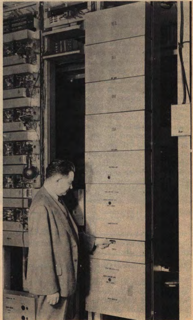
TYPE-K CARRIER SUPPLY BAY
