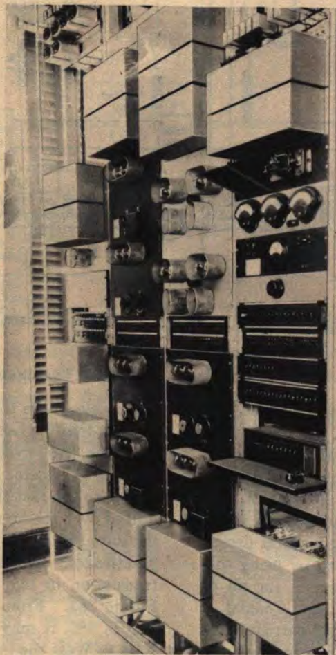
TERMINAL EQUIPMENT OF TYPE-C CARRIER SYSTEM
