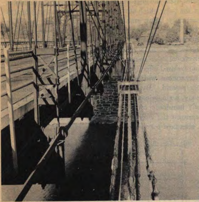
STANDARD TOLL CABLES AND COAXIAL CABLE (SECOND FROM LEFT) INSTALLED ON BRIDGE
