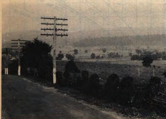
TOLL CABLE IN BACKGROUND— 12-INCH SPACED OPEN WIRE LINE IN FOREGROUND
