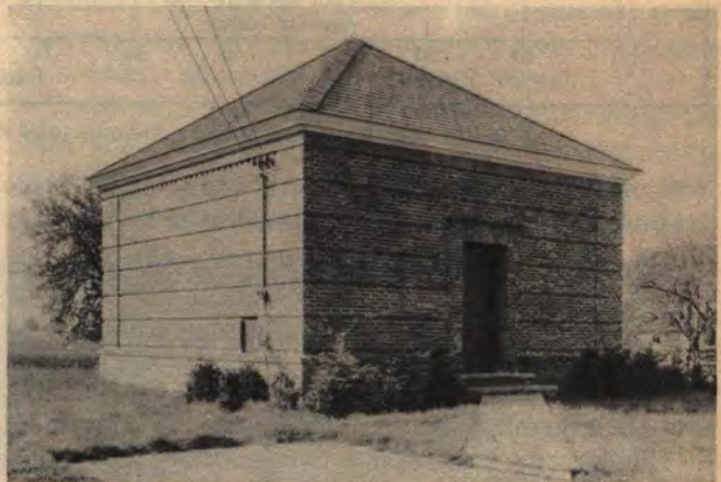
AUXILIARY CABLE CARRIER REPEATER STATION
