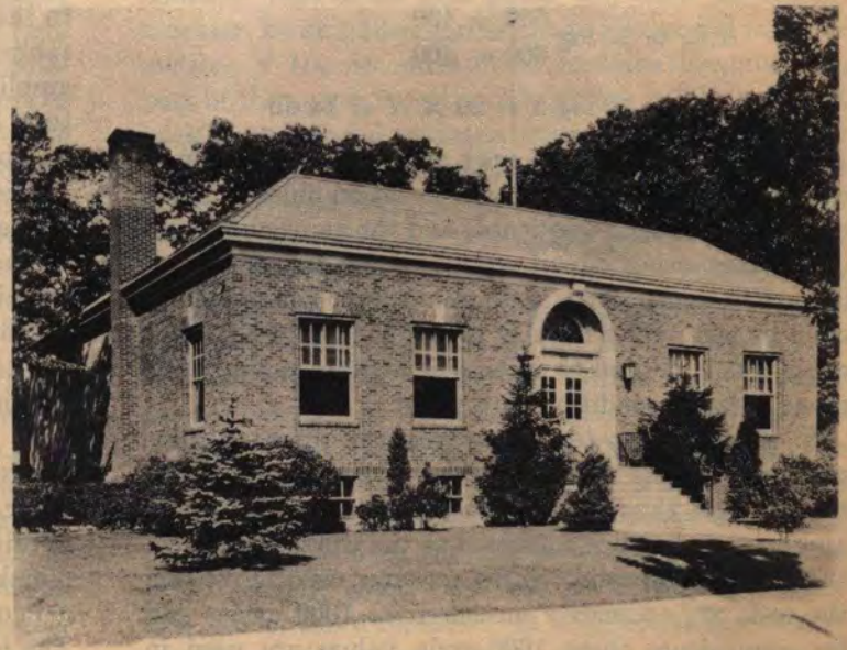
CABLE REPEATER STATION AT WAUKEGAN, ILLINOIS
