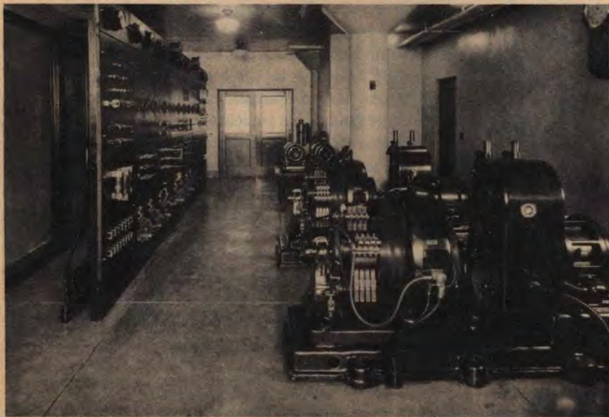
TYPICAL REPEATER STATION POWER PLANT
