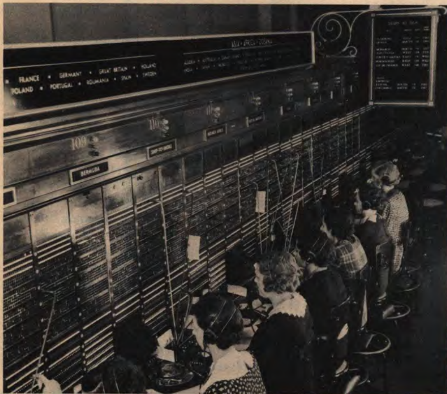
OVERSEAS TOLL SWITCHBOARD
