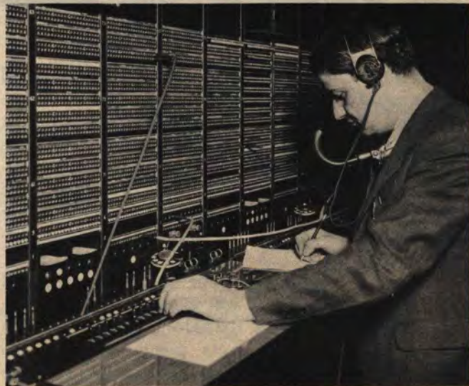
No. 8 TEST AND CONTROL BOARD
